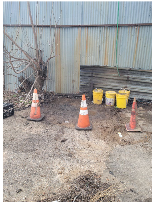
Stained surficial soil around DRUM-01 contained and area secured
