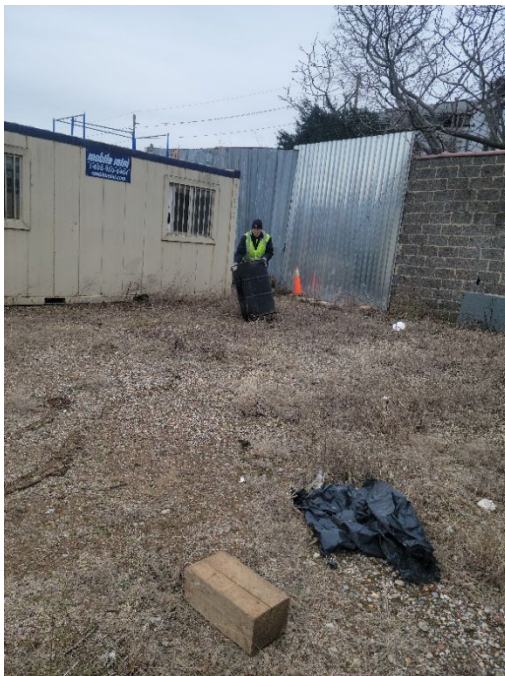
Removal of drums from storage area on Block 331
