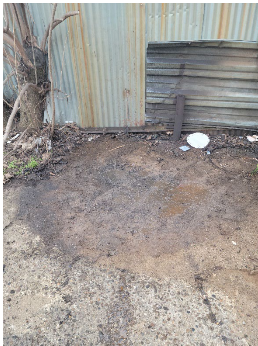
Stained surficial soil around DRUM-01 scraped off concrete and removed
