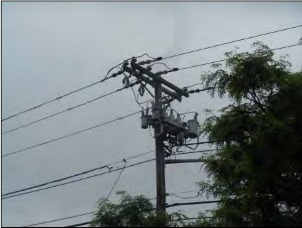
View of AOC 7.
