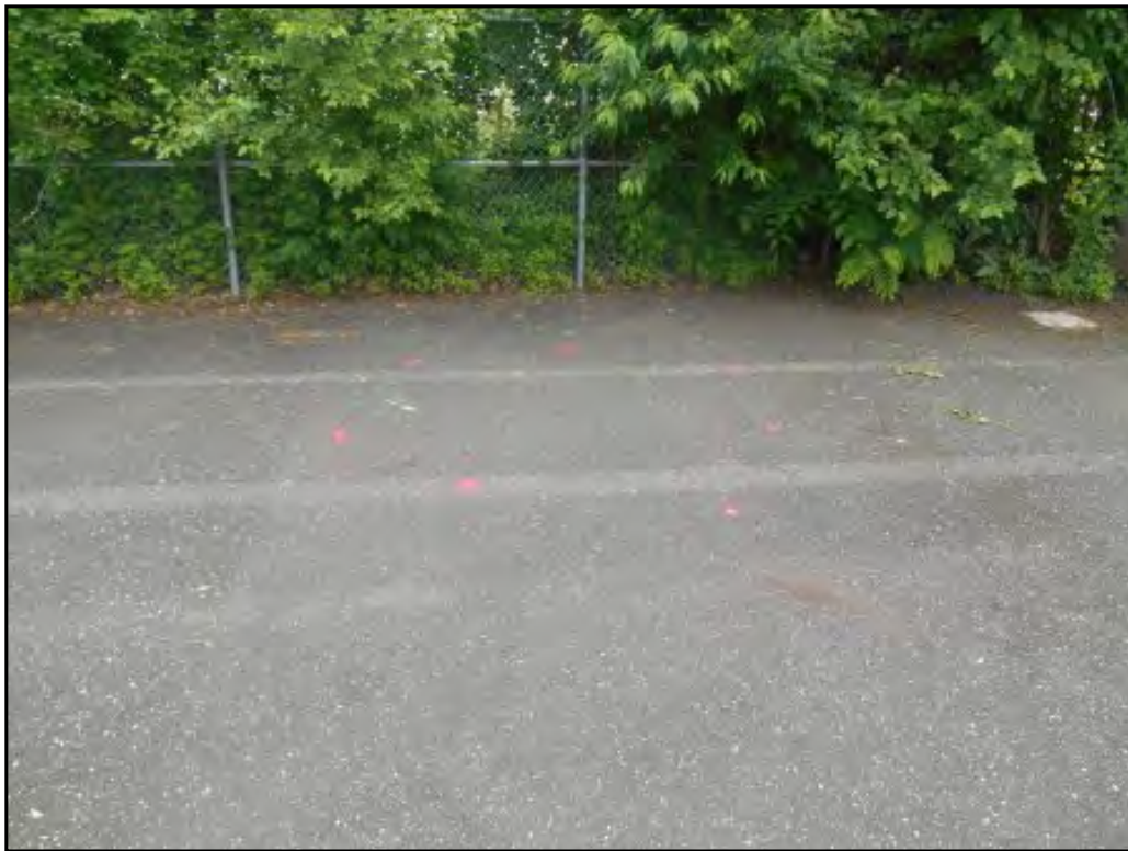
View of AOC 5 on the northeastern corner of Block 14, Lot 29.
