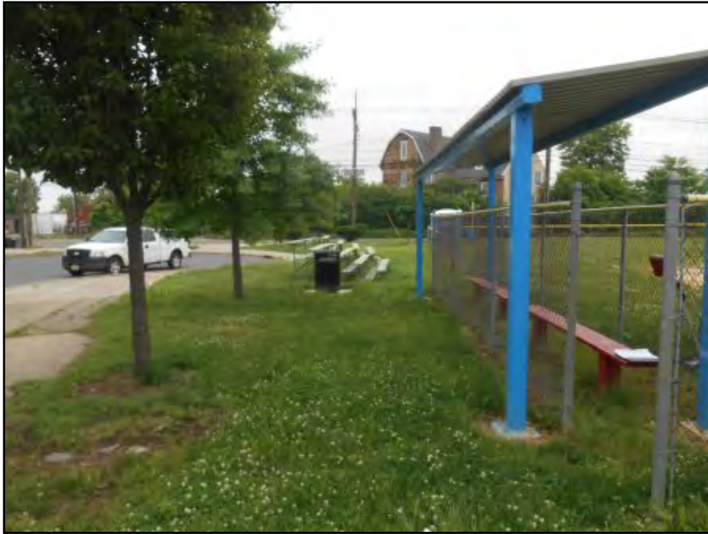
Western boundary of Block 12, Lot 1.
