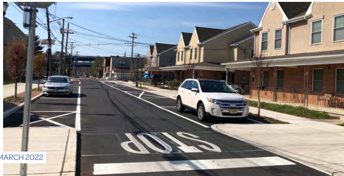
Newly paved streets compliment new construction homes on the 700 block of N. 2nd Street
