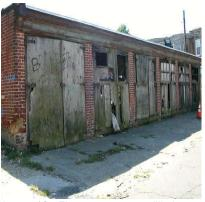
Image 18. These garages are filled to their roofs with garbage, creating a health hazard. The structure is crumbling and poses a safety risk.
