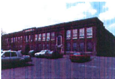
Top: View of Yorkship School from the Collings Road recess yard/parking lot.
