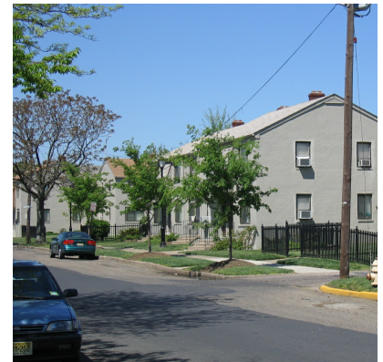
Image 9. Liberty Park Apartments (formerly Everett Gardens Apartments) have been recently renovated.
