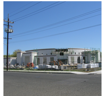
Image 17. First Nazarene Baptist Church's new sanctuary construction site.
