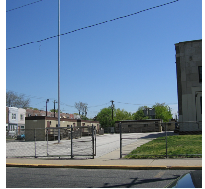
Image 20. Sumner School's trailer annex facilities.
