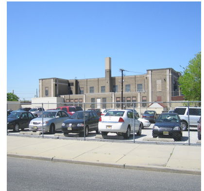
Image 3. Parking facilities behind Charles Sumner Elementary School.
