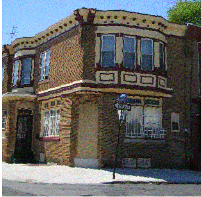
Image 23. A recently renovated house.
